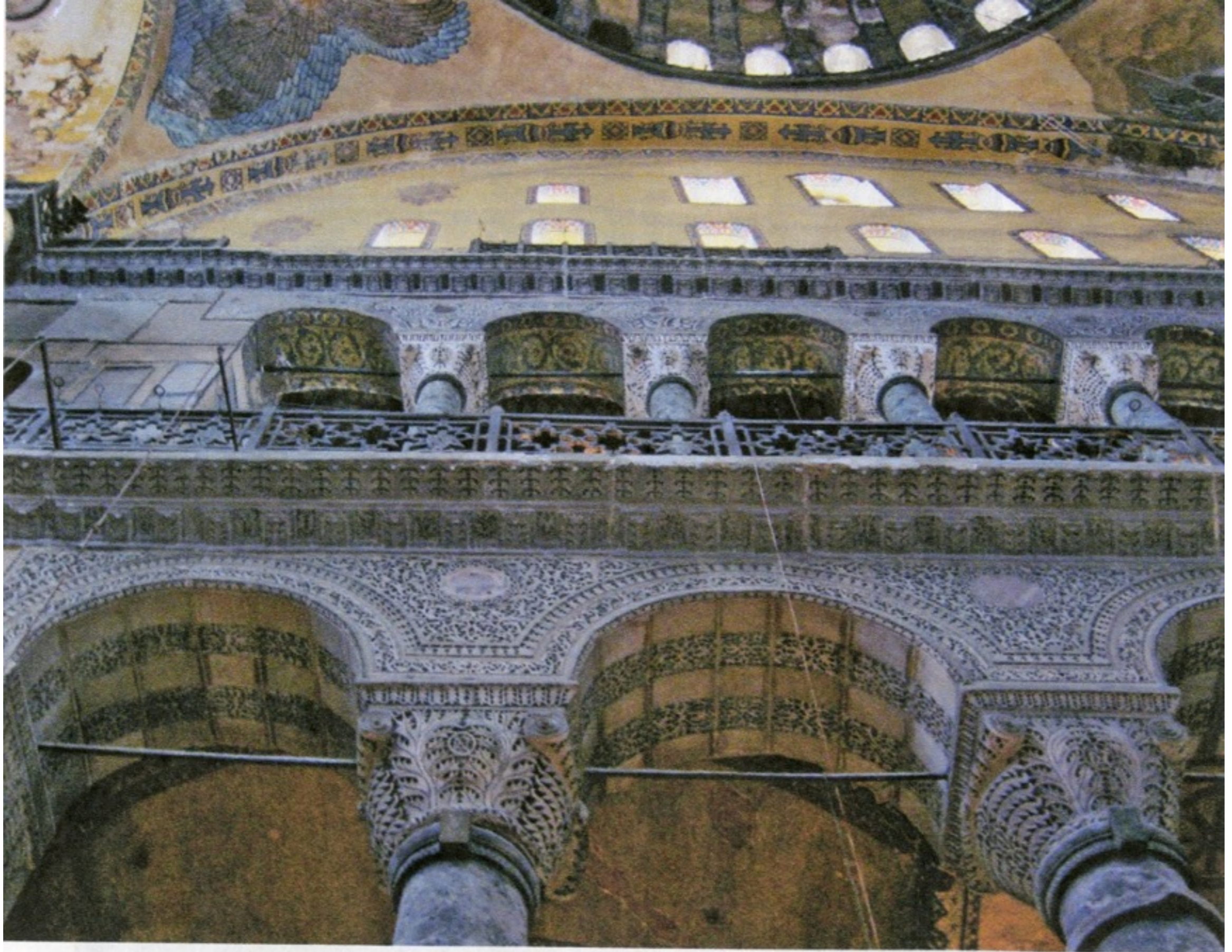
Figure 6.2-7 Constantinople. Hagia Sophia, interior elevation, showing misalignment of columns on the second level.
