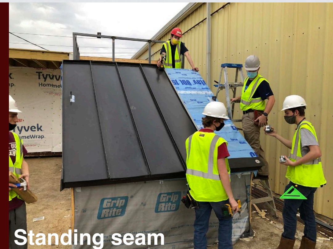
Head-wall & rake-edge flashing
