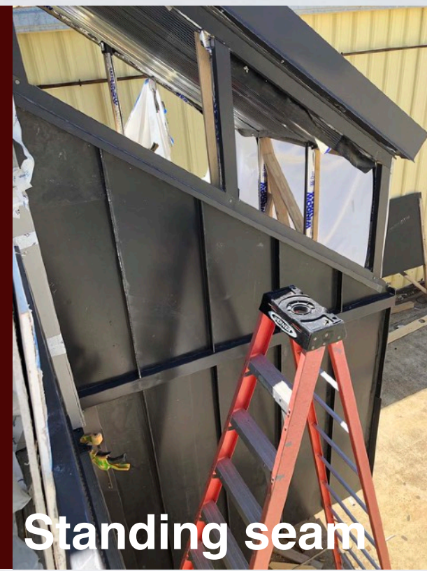
Prep for reverse board & batten
