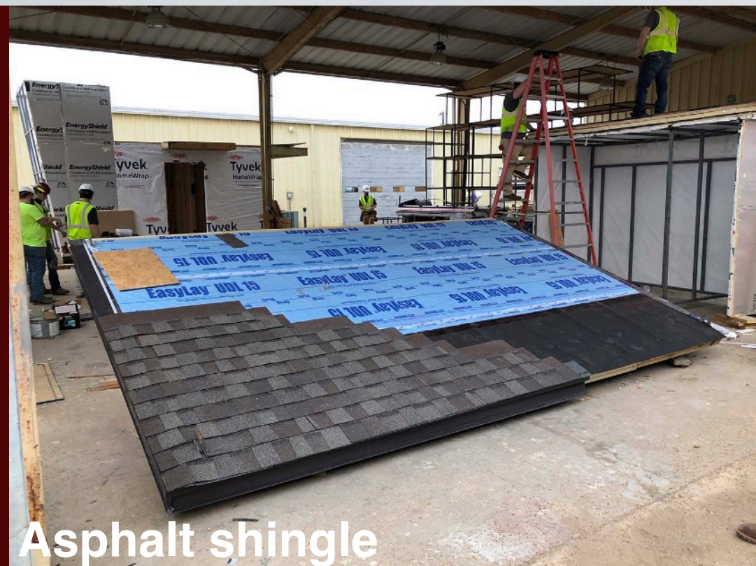
Good drip-edge flashing
