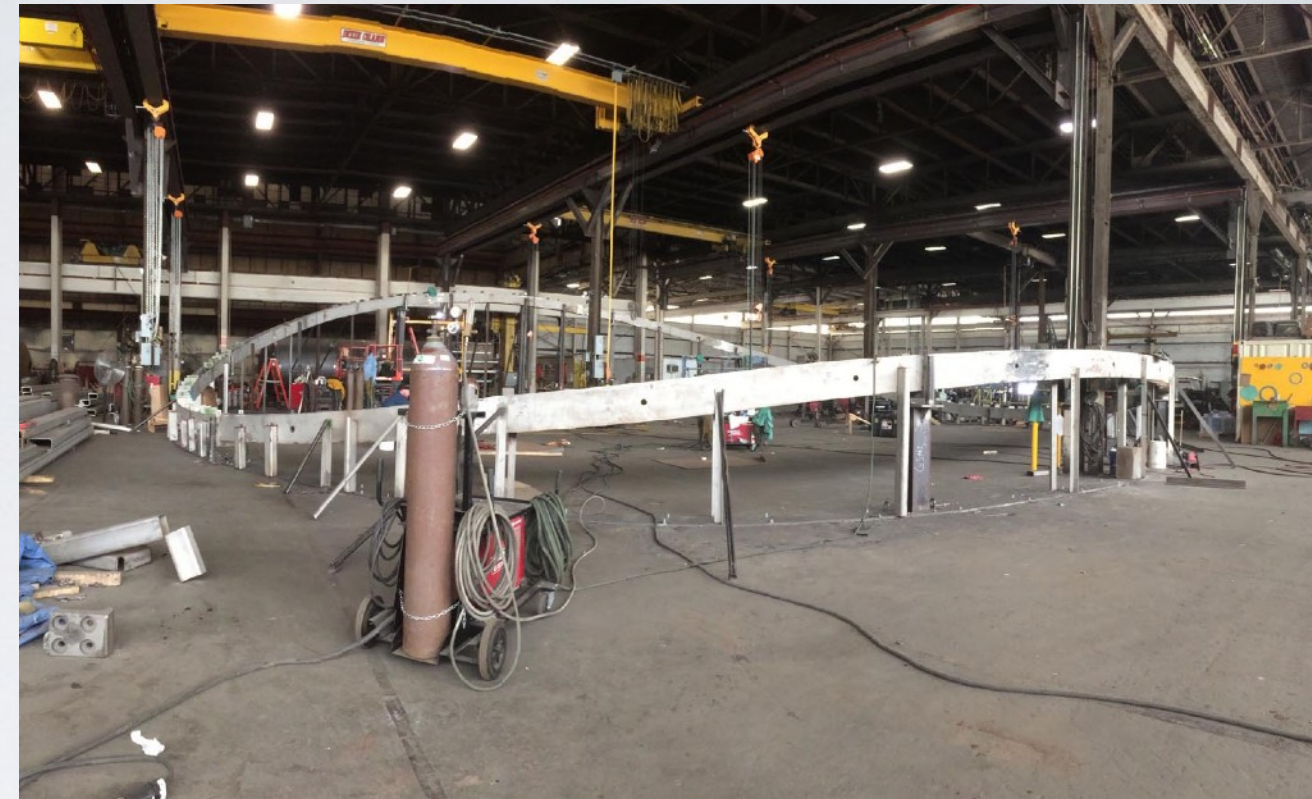
Making the giant Ring Girder
