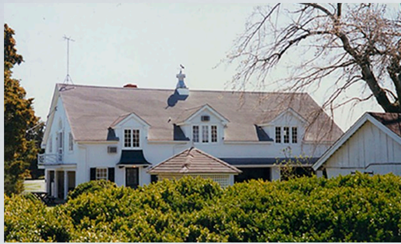
Renovation of a Carriage House, Oxford MD Architect
